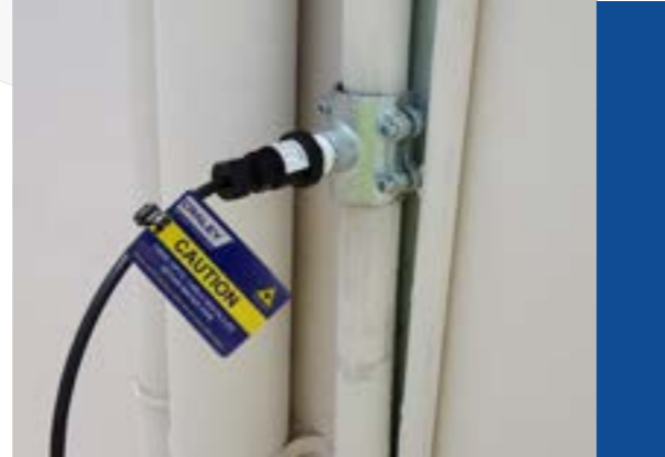
CRALEY Fibre Final Fitting Installation
